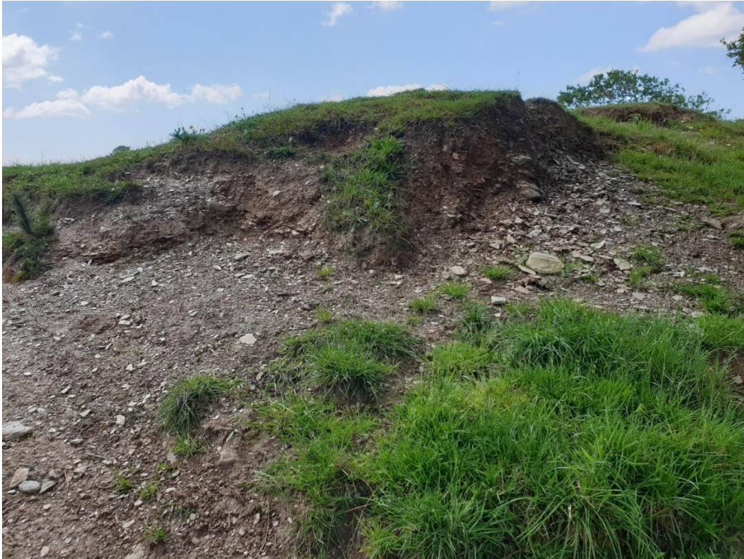
Fig 15 Priority erosion area P4 facing south-west, showing the exposed core of the rampart.
