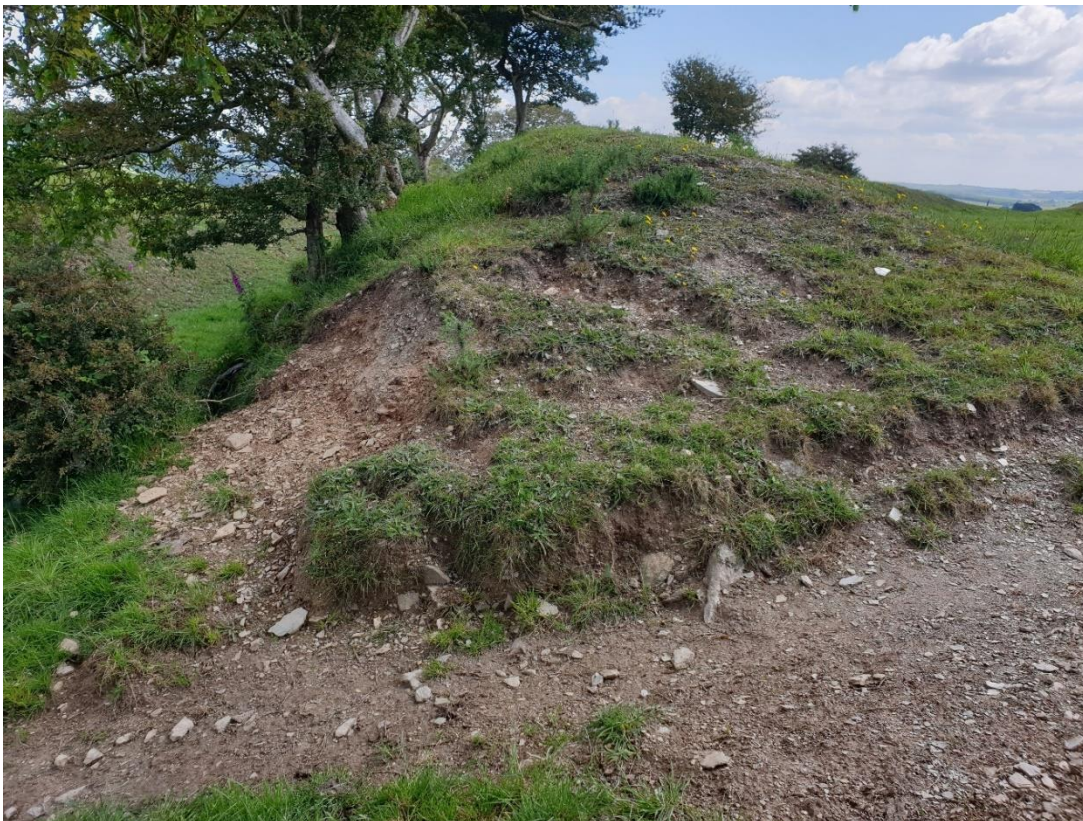
Fig 16 Priority erosion area P4 facing south-west, showing the exposed core of the rampart.
